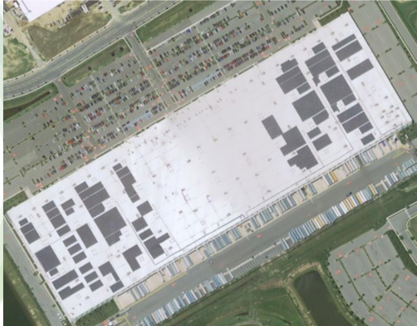
Warehouse with solar panels on roof
